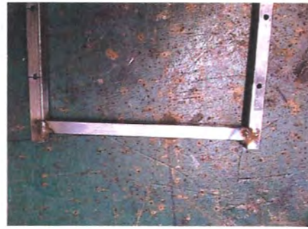
As a result, I had to MIG weld the mild steel bar to the legs
